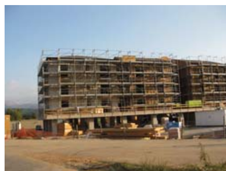
New facilities under construction in Abruzzo
